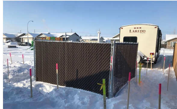
Fencing around the well site in the Brennan playground
