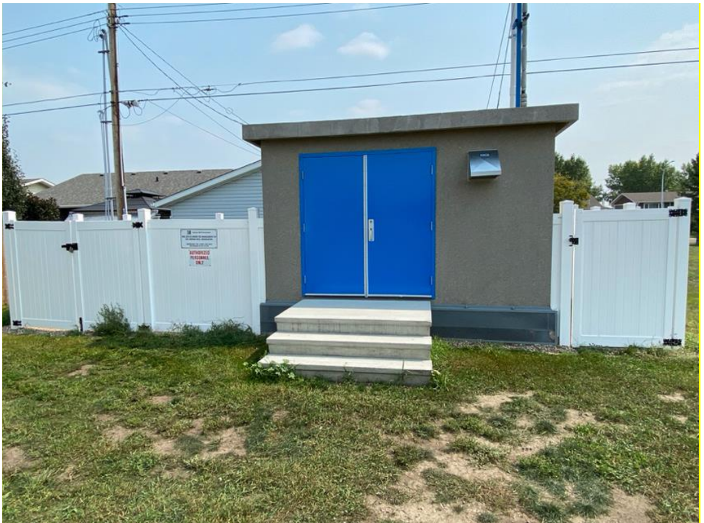
Final AMMS installation at the historic gas well
